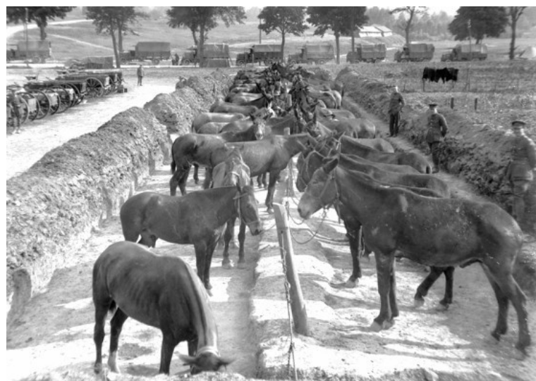
Horse lines near Amiens showing bomb protection. AWM Photo: EO2432
